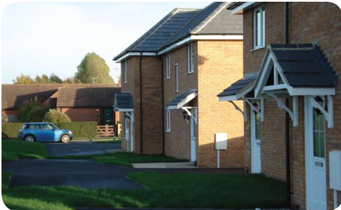
New homes built by the Local Housing Company in Tydd St Mary, South Holland (image courtesy of South Holland District Council)
