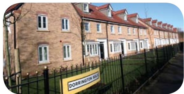
New development in Liverpool, Dorrington Walk (reproduced with kind permission of Liverpool City Council)
